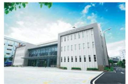
LESSO Research Institute & Testing Center
