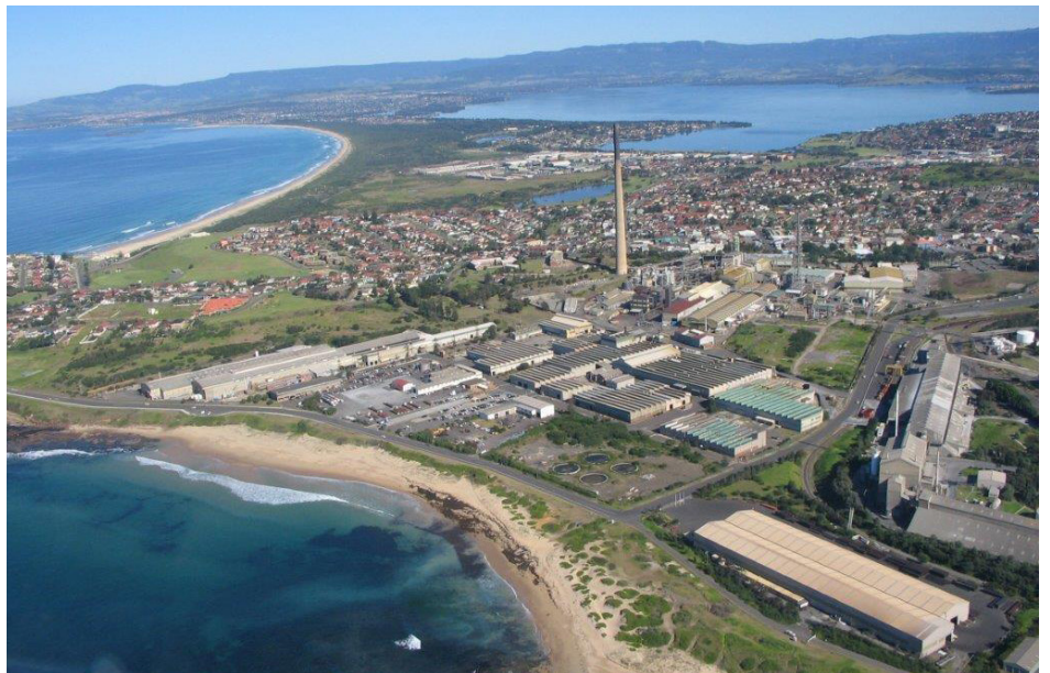
MM Kembla's Australian manufacturing facilities at Port Kembla.
