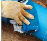
2. Clean the exterior of the pipe before applying the lubricant
